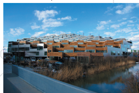
BIG, Mountain Dwellings , Copenhague, 2005 (construction en cours)
